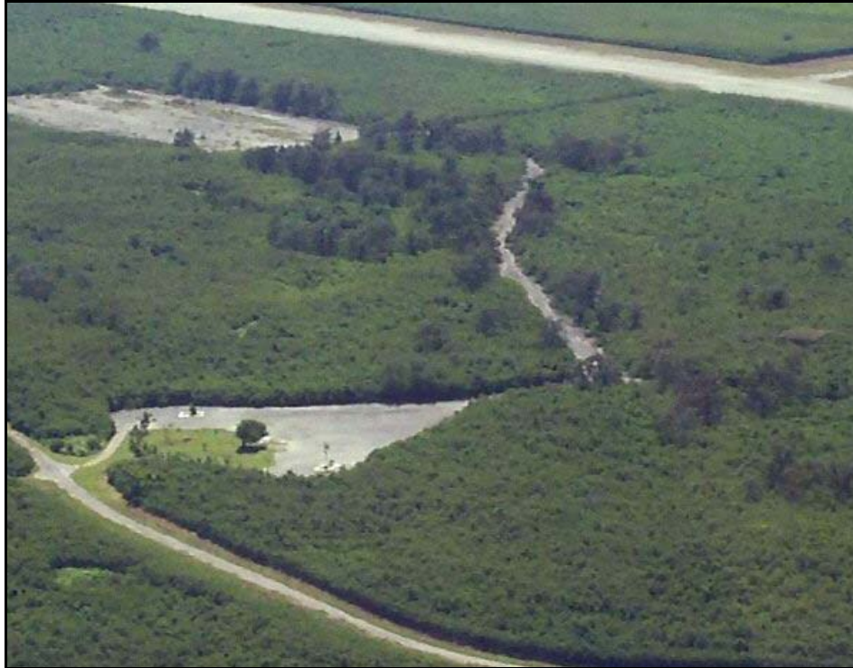
Figure 13.1-7. An Aerial View of the National Historic Landmark and Bomb Pit Enclosure (Lower Left Side of Photo)
