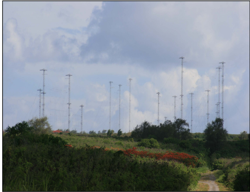
Figure 12.1-4. Antenna Array of Mariana Relay Station
