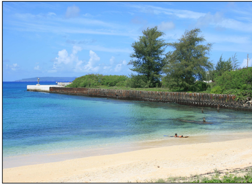
Figure 12.1-5. Tinian Harbor, East Quay, Looking Southwest
